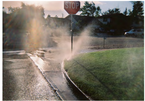
High pressure and overspray onto a street
