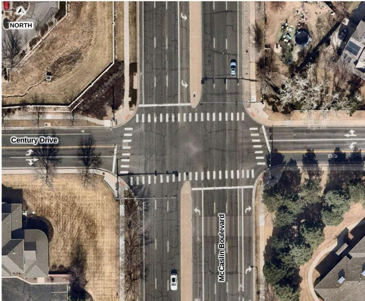
Century Drive & McCaslin Boulevard (#2)
