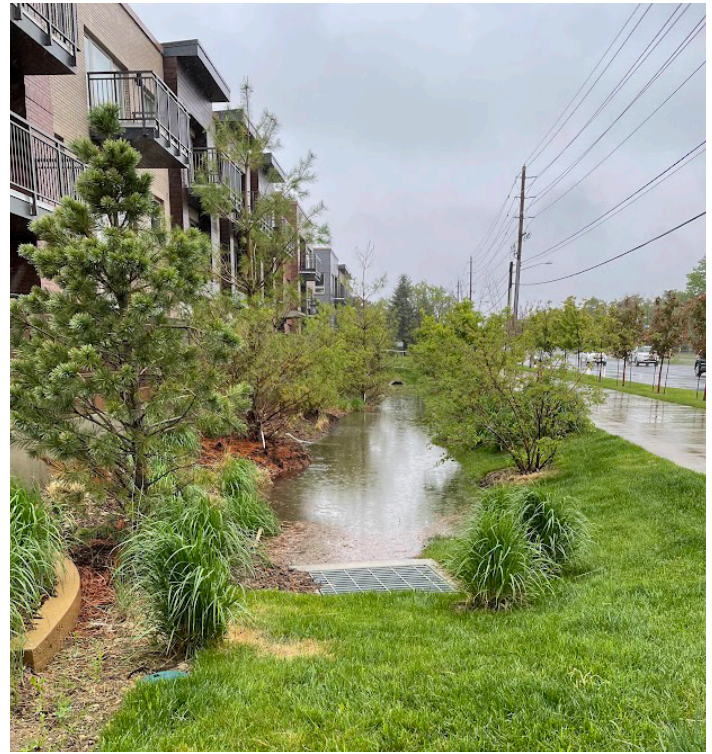
Photograph BR-2. Bioretention system treating urban stormwater during runoff event. Photo: Wright Water Engineers.
