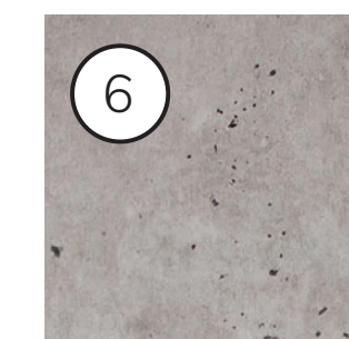
Cast in Place Concrete - Smooth finish
