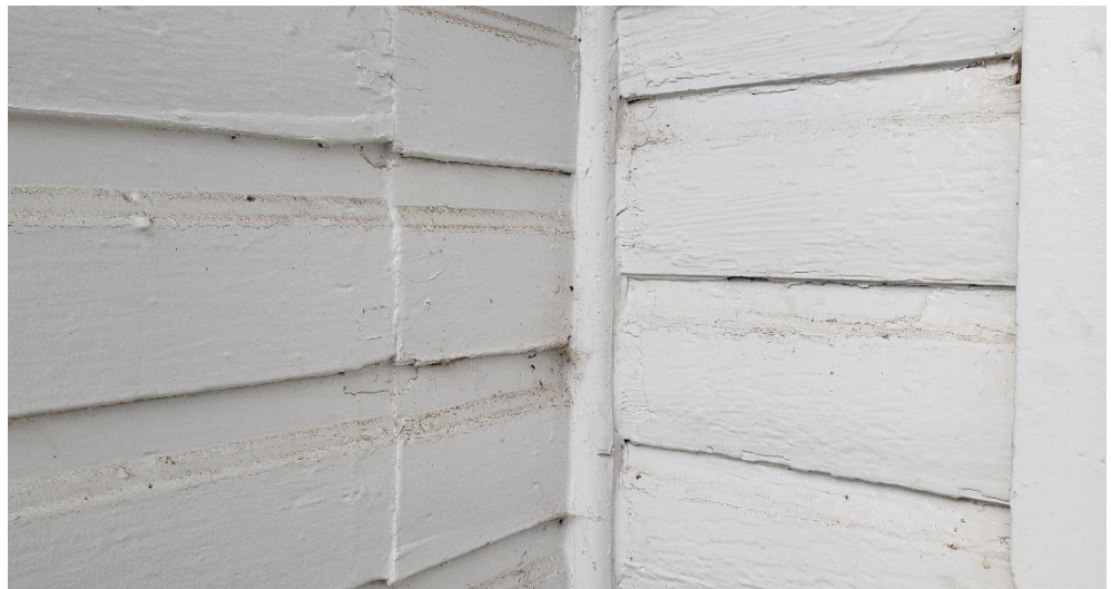
Original wood siding (left) next to the dutch-cove profile used in later additions (right).
