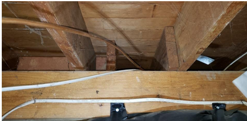
Spliced floor joists on a support beam in the 1941 addition.
