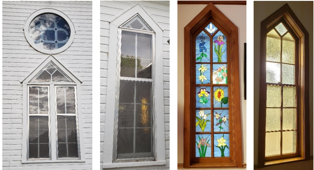
Typical windows found on the earliest parts of the church.
