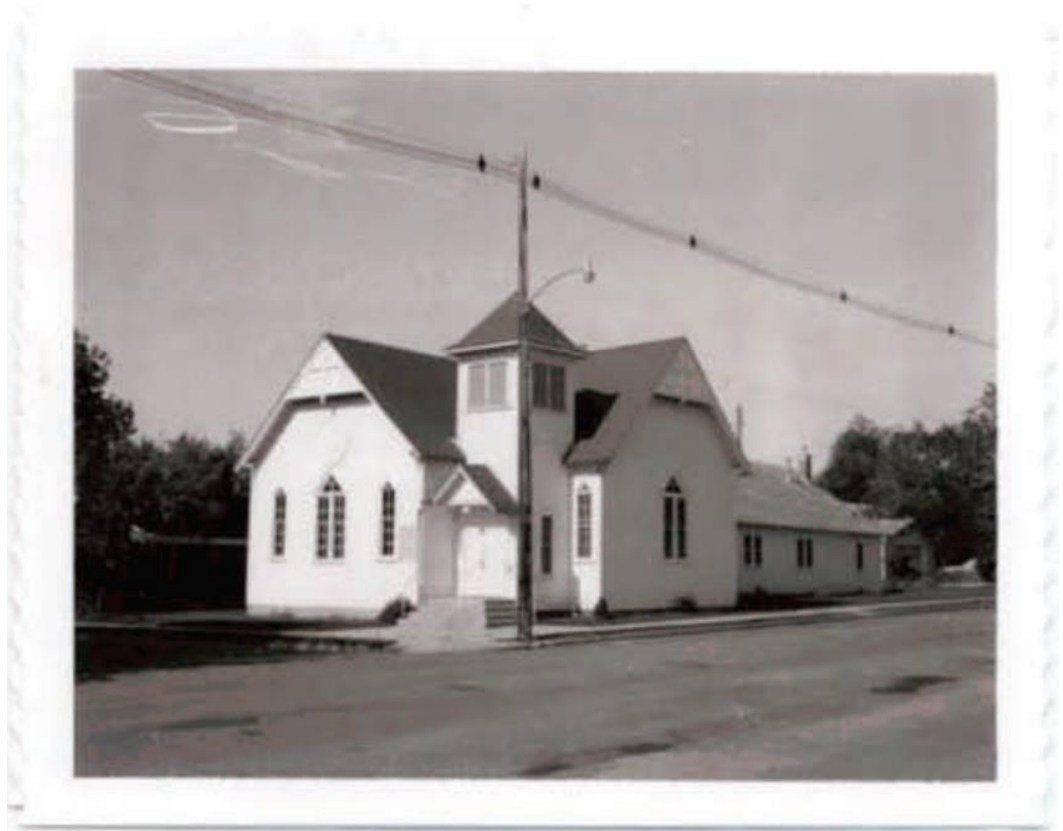
Circa 1941 view of from the northeast. The 1941 addition is present at the rear of the church.
