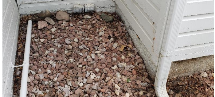
Foundation of the 2000 addition is exposed above grade while the older foundations are not.
