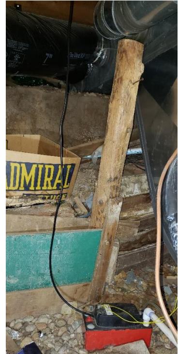
Various materials have been used to brace the cut soil.
