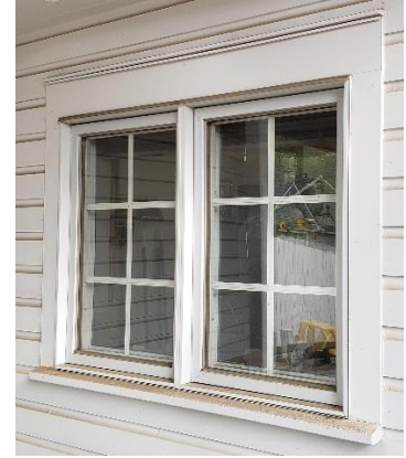
2000 addition paired windows.
