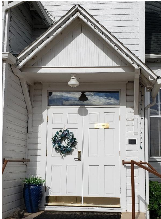
Front entrance doors and transom in 2024.
