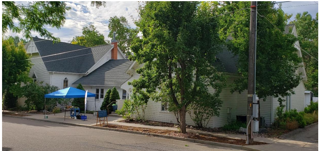
2024 view from the northwest. The 1941 addition is visible while the 2000 addition is mostly obscured by mature trees.
