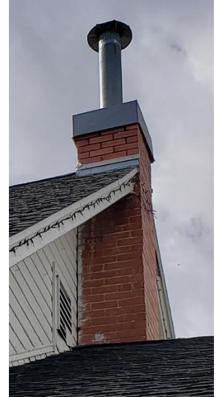
Brick chimney in 2024.
