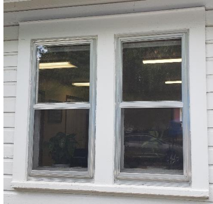
1941 addition paired windows.
