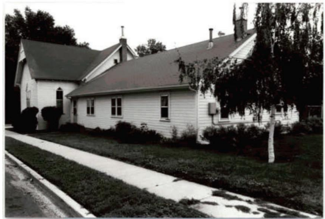
Circa 1941 view of from the northwest. The 1941 addition is present at the rear of the church.
