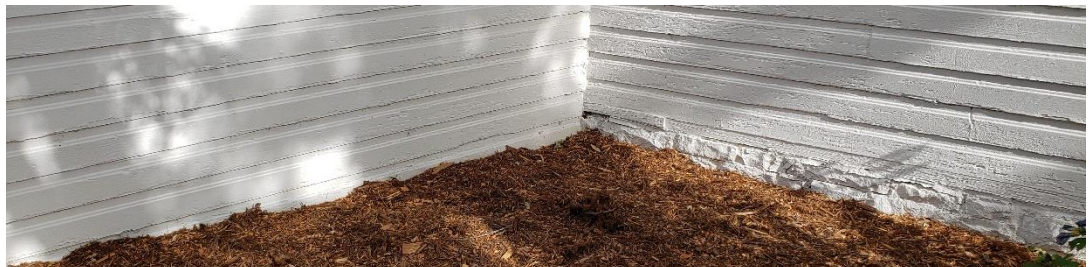
The original stone foundation is seen from the exterior on the right. The south addition on the left does not have an exposed foundation above grade.
