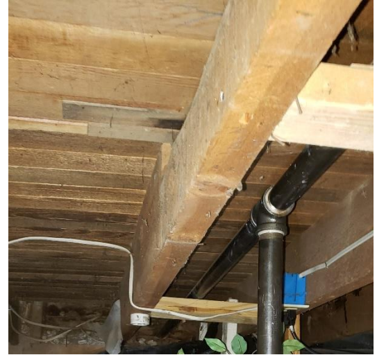
Original construction floor framing & underside of flooring seen in the basement.
