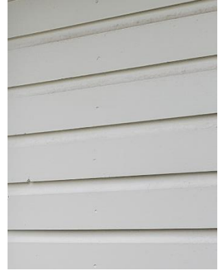
Dutch cove profile siding used in the 2000 addition.
