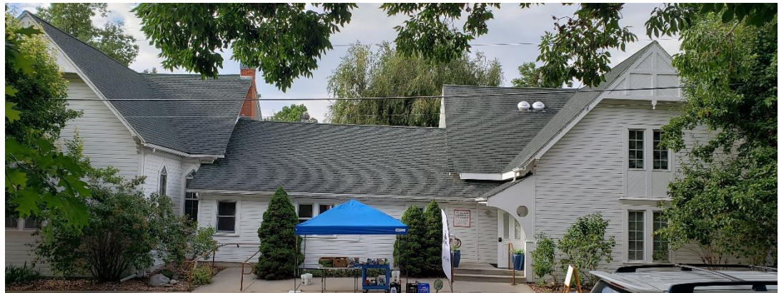
An asphalt composite shingle roof covers all aspects of the building.
