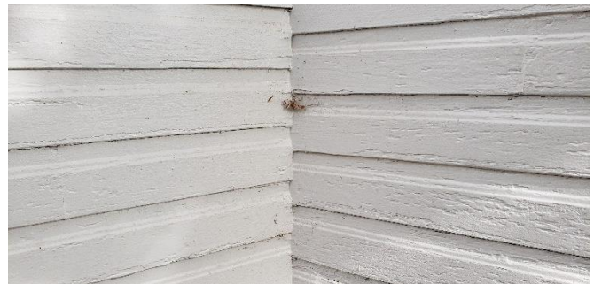
Original shiplap siding where the south addition meets the original church structure.
