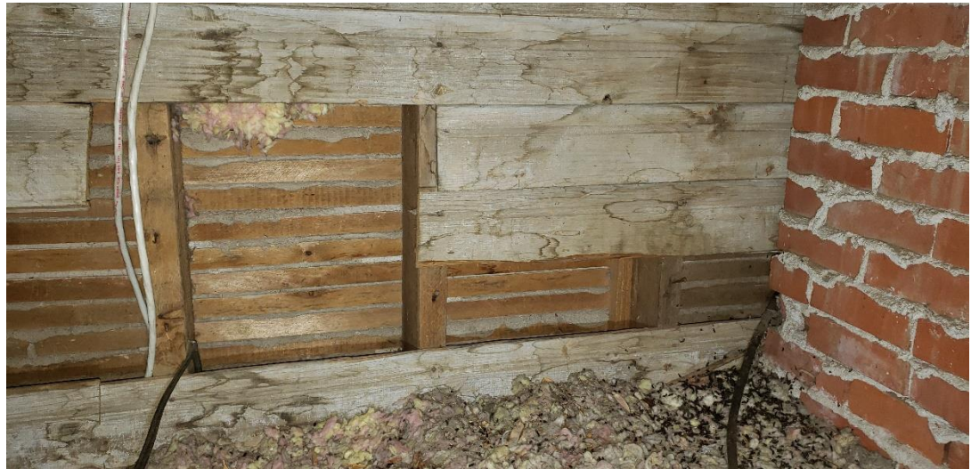
Original west wall as seen in the attic of the 1941 addition.
