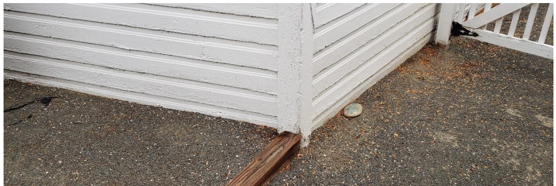
Finish materials run beneath grade all around the south altar bay.
