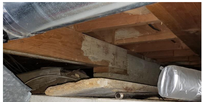
Floor framing and grade beam of the 1941 addition.
