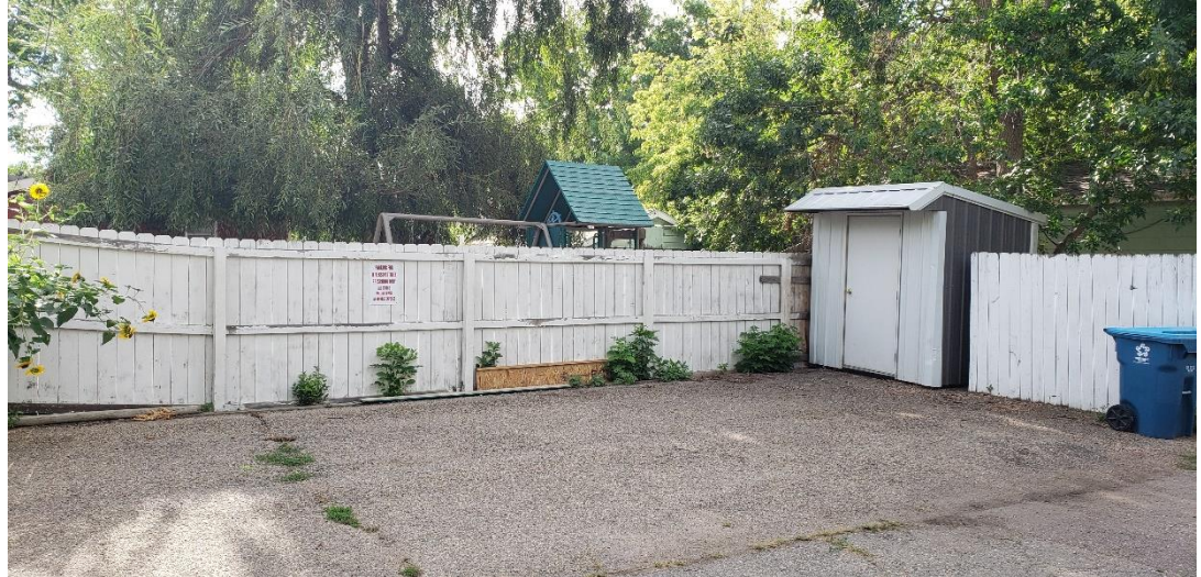
Asphalt parking area along the west alley behind the preschool.
