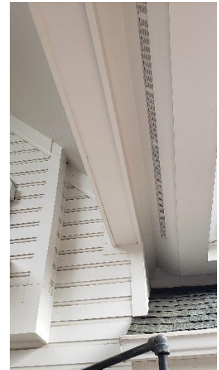
Soffit venting at the 2000 addition roof eaves.
