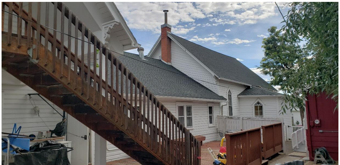
2024 view from the southwest in the yard behind the preschool. The addition on the south of the original church is visible.
