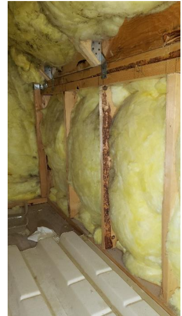
Roof framing of the 2000 addition supported by a pony-wall.
