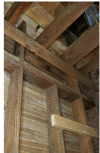
Wall framing of the bell tower is likely similar to that of the original church.
