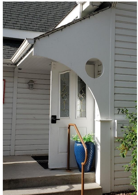
Several matching exterior light fixtures appear to have been added in 2000.
