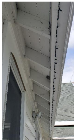
1941 addition rafter tails.
