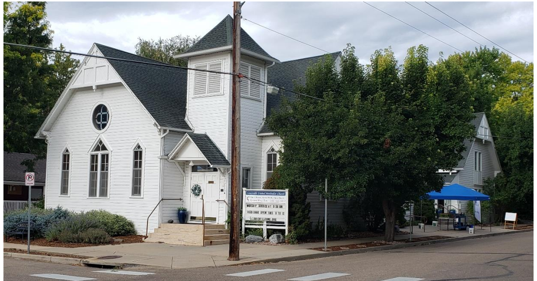
2024 view from the northeast. The 2000 addition is visible in the background. The 1941 addition is obscured by mature trees.
