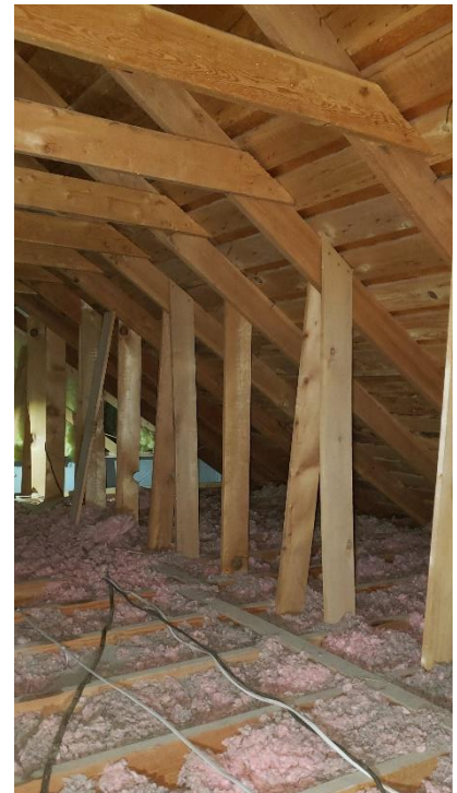
Roof framing of the 1941 addition.
