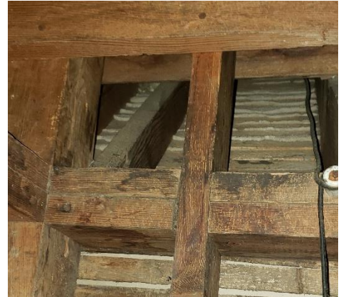
Original roof framing is only partially visible from within the belltower. Original lathe and plaster ceiling can be seen.
