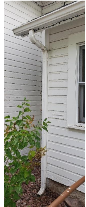
K-style gutter and 2x3 downspout typical of entire building. Not all downspouts have extensions.
