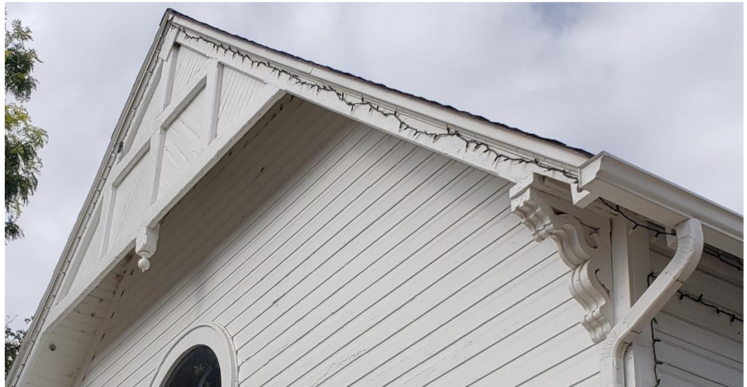
Gable end barge boards, pendants, and brackets found on the original construction and 2000 addition.
