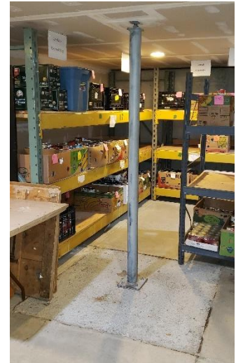
Steel column and footing in the 2000 basement.
