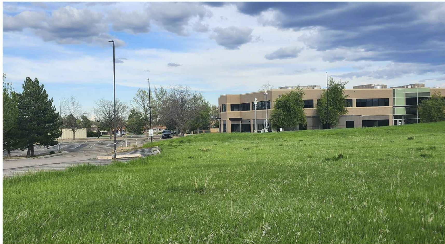
EXISTING CONDITION View east-southeast from Century Place
