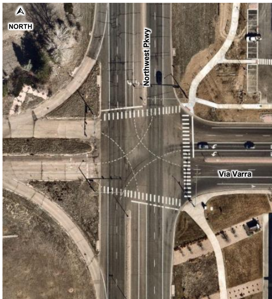
Via Varra & Northwest Parkway (#3)
