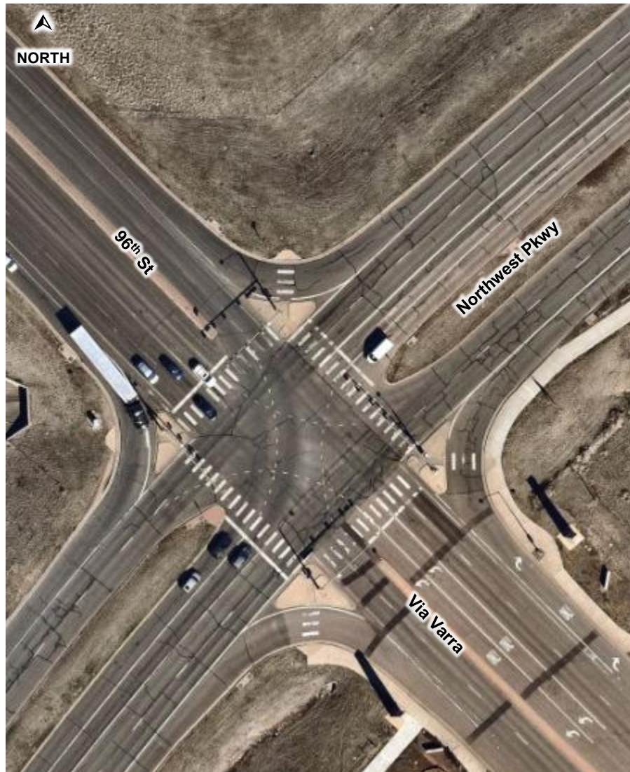
96 th Street/Via Varra & Northwest Parkway (#2)
